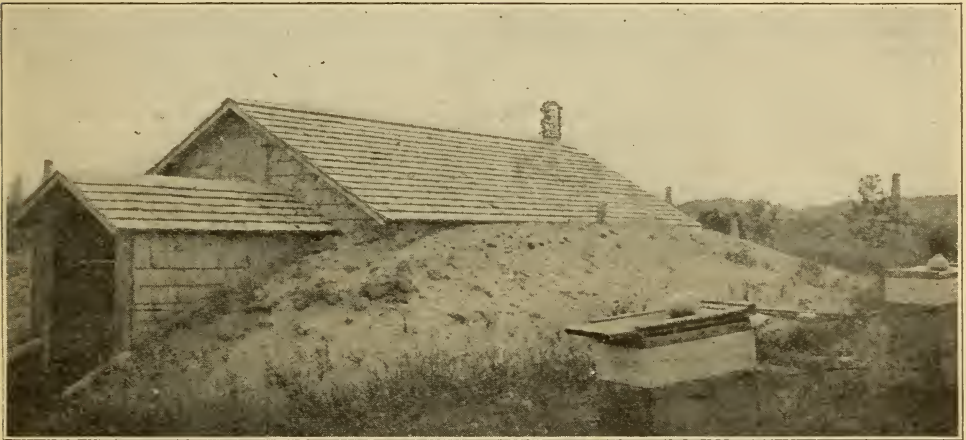
FIG. 4.—This cellar belongs to L. C. Gordon, of Bellaire, Mich. According to David Running's idea the roof should have extended over the side embankment. But these embankments are made up of sand that dries out very quickly; and in spite of the fact that it is not covered, it makes a good insulator. Mr. Gordon once told the author that in this 12x20-foot bee-cellar the preceding winter he wintered 151 colonies without the loss of a colony. This cellar has the ventilation recommended by Mr. Running.
